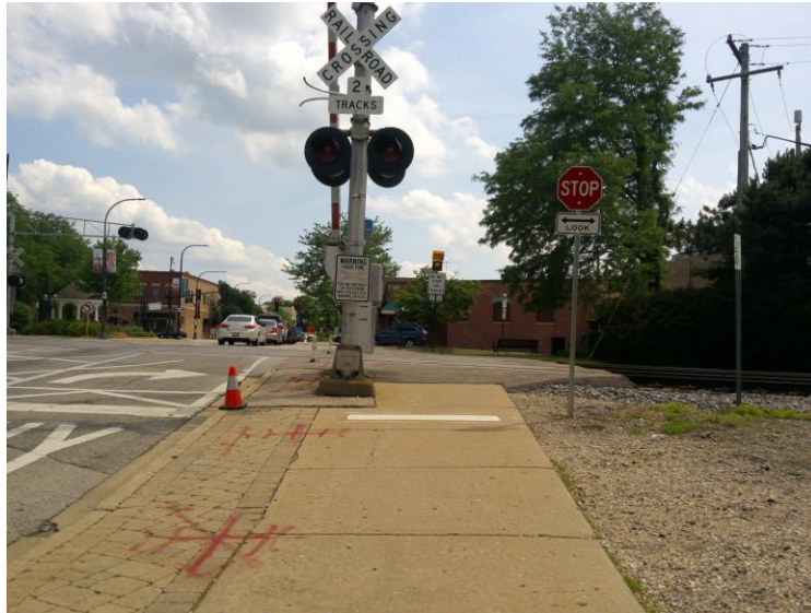
Figure B: Photograph showing the Hough Street Crossing facing south.
