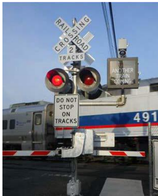
Figure E: Warning Sign for Another Train Coming
